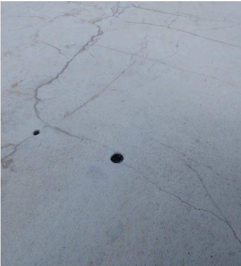
Figure 4 Example of incorrect thickness resulting in failure
