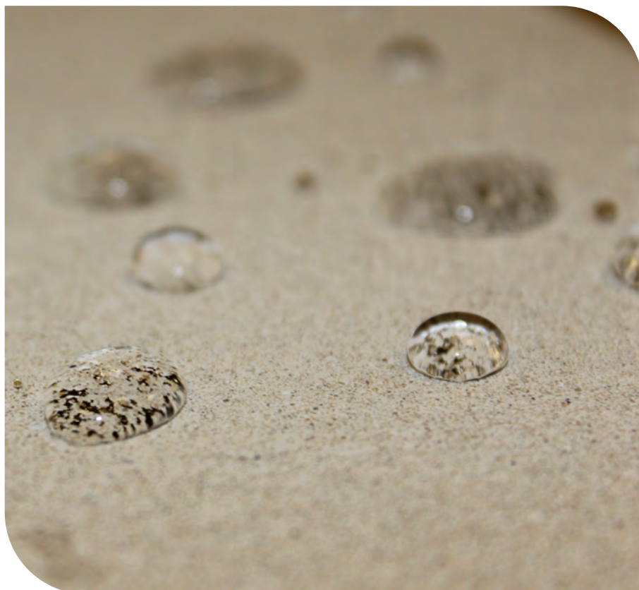
ABOVE: Surface sealant applied to facing coat.
