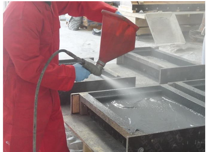
Application of facing coat
